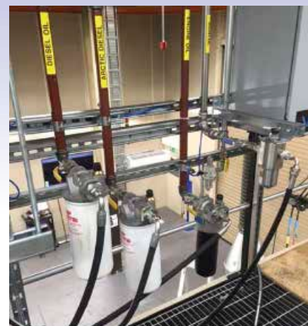
LMP 210 in-line filters and MPS Spin-on for diesel, engine oil, adblue fluid
